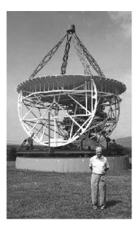
Figure 1.3 Grote Reber's home-built backyard radio telescope (photo courtesy of NRAO).
