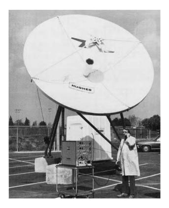
Figure 1.6 A 4.5-m earth station capable of telephone service (circa 1977).
