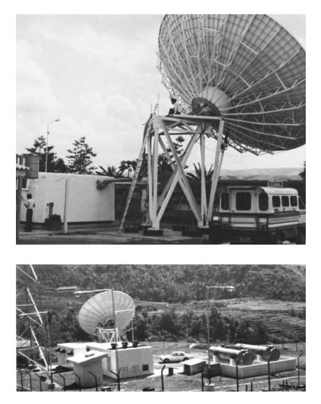
Figure 1.5 Palapa A light-traffic earth station (10-m antenna) in Indonesia.
